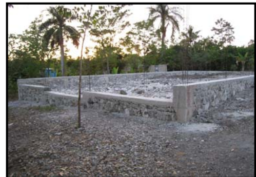
Marchasse Church building foundation
